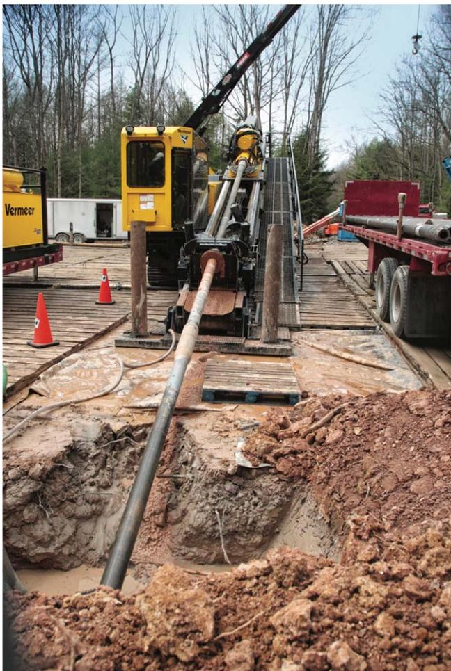
**Figure 2. 22 bores in total were completed on the Cedar Station Upgrade project using horizontal directional drills.**
