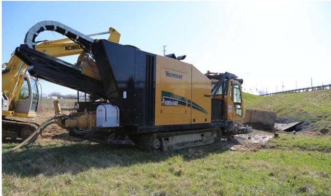
**Figure 1. Minnesota’s sandy soils meant crews would have to take extra precautions to maintain the integrity of the bore hole, mitigate sinkholes, and minimise any inadvertent returns.**
